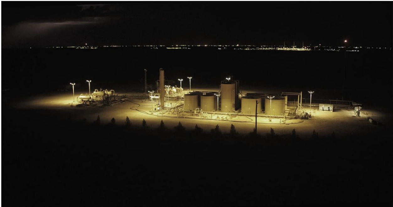
Photo #3. Apache Corporation tank battery near Balmorhea, Texas, using night sky friendly lighting. The Diamond Cryo Complex (photo #4, below) is visible on the horizon to the top, right.
