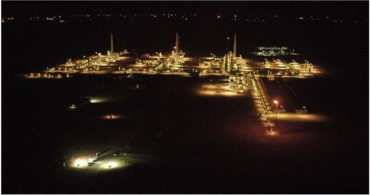
Photo #4. Apache Corporation Diamond Cryo Complex near Balmorhea, Texas, using night sky friendly lighting.
