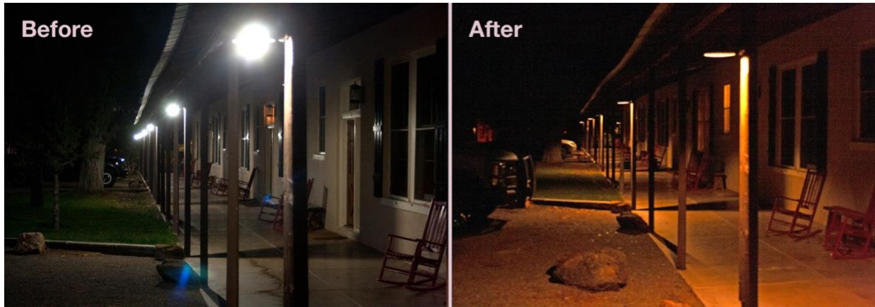
Photo #2. Lighting at the Hotel Limpia in Fort Davis, Texas. Partially shielded “cool-white” bulbs (left) replaced by fully shielded “warm-white” ones (right). Hotel maintenance staff report routinely picking up the former from the ground in the morning after guests removed them due to harsh white light shining into their rooms.
